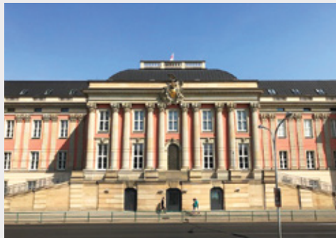
Landtag of Brandenburg, Germany - GMA Garnet™ ClassicCut 80 was used to manufacture custom designed fixing brackets for the parliament extension.
