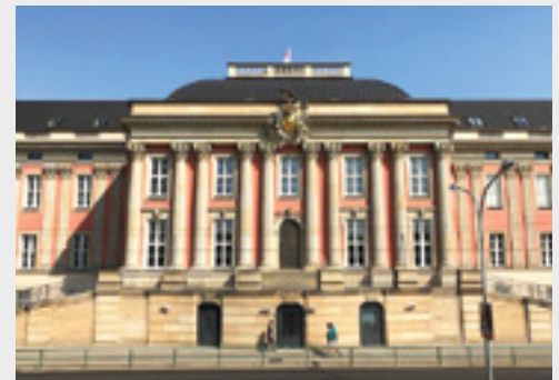
Landtag of Brandenburg, Germany - GMA Garnet™ ClassicCut80 was used to manufacture custom-designed fixing brackets for the parliament extension.
