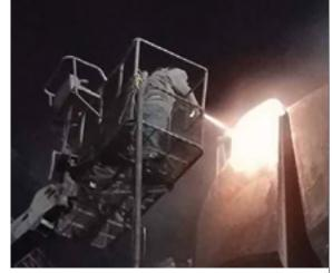
\*Production and consumption rates may vary based on nozzle size, pressure at the nozzle, standoff distance, abrasive metering, equipment quality, surface type, coating type and thickness. The blasting rates are achieved by setting the nozzle pressure to operate within the range of 95 psi – 100 psi. GMA will work with you to produce optimum performance on blasting jobs, reducing time and cost, and producing the best surface result for any coating.
