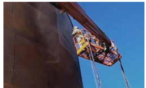
*\*Production and consumption rates may vary based on nozzle size, pressure at the nozzle, standoff distance, abrasive metering, equipment quality, surface type, coating type and thickness. The blasting rates are achieved by setting the nozzle pressure to operate within the range of 95 psi – 100 psi. GMA will work with you to produce optimum performance on blasting jobs, reducing time and cost, and producing the best surface result for any coating.*
