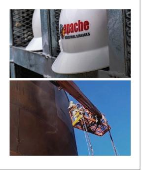
\*Production and consumption rates may vary based on nozzle size, pressure at the nozzle, standoff distance, abrasive metering, equipment quality, surface type, coating type and thickness. The blasting rates are achieved by setting the nozzle pressure to operate within the range of 95 psi – 100 psi. GMA will work with you to produce optimum performance on blasting jobs, reducing time and cost, and producing the best surface result for any coating.
